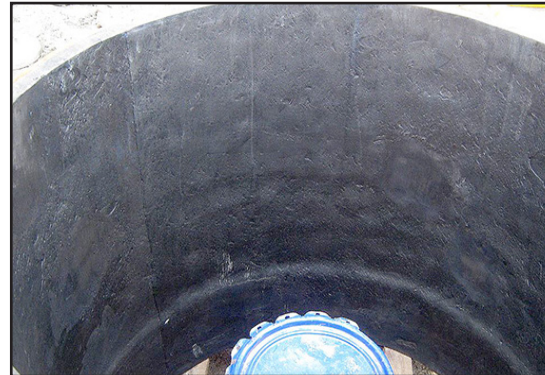
Rubber surface is prepared by roughening with flapper wheel.
